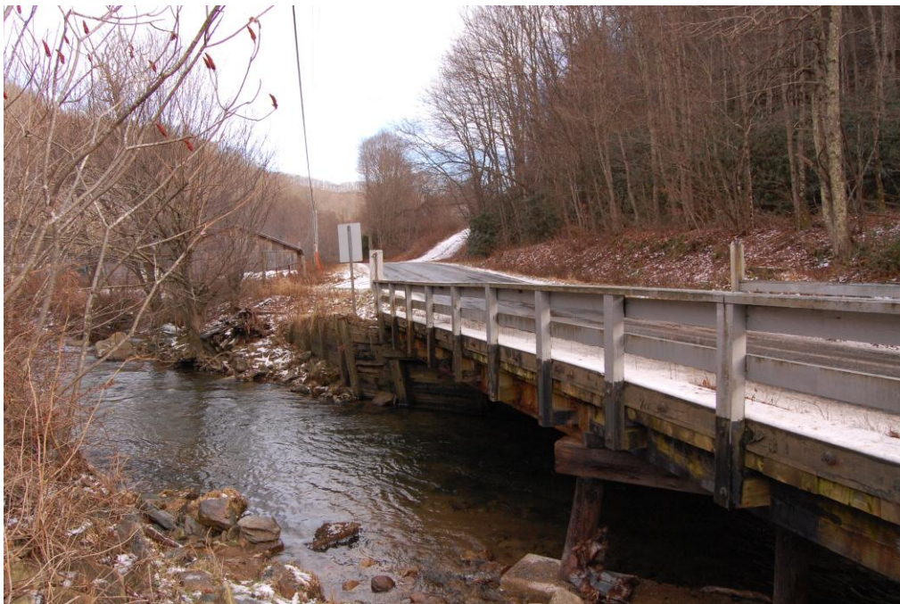
Figure 3: View to the east-southeast along Big Horse Creek Road and Bridge No. 66
