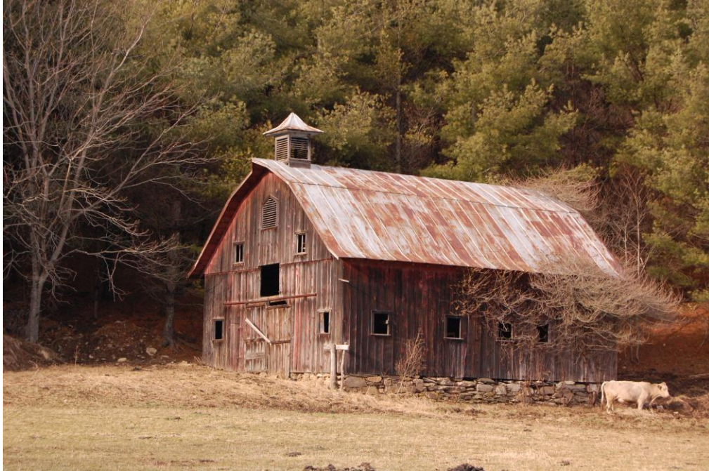
Figure 5: Barn at Lee Little Barn and Outbuildings, view toward the north-northwest
