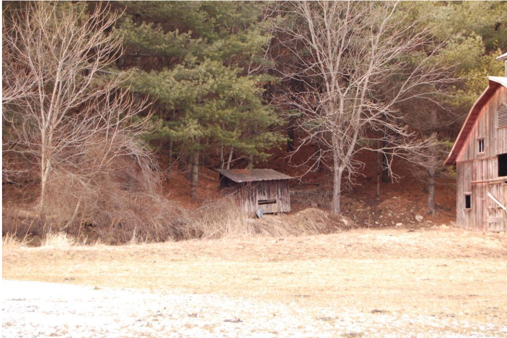
Figure 1: Pig house and Barn at Bridge No. 66, view to the north-northwest
