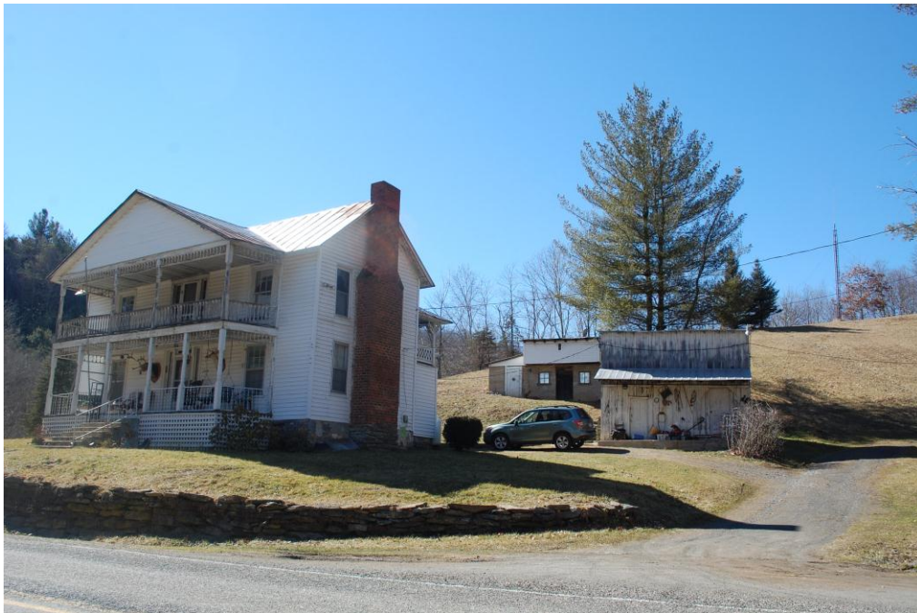
Figure 14: The Isham Goss Farm (AH 106) includes an I-house, cellar building or apple house, and other outbuildings
