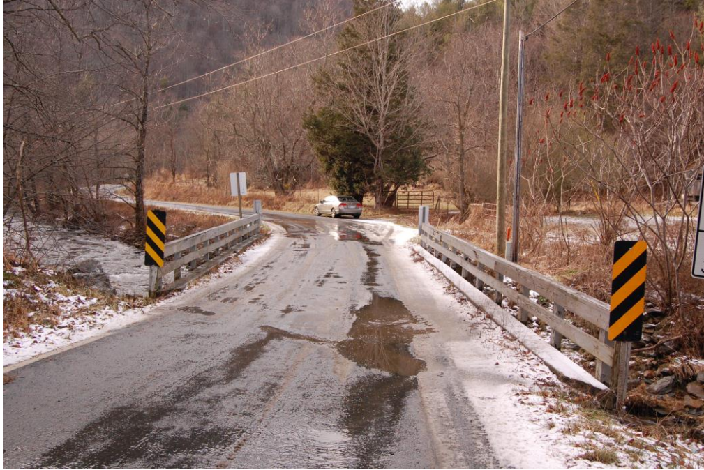
Figure 4: Bridge No. 66 along Big Horse Creek Road, view to the west
